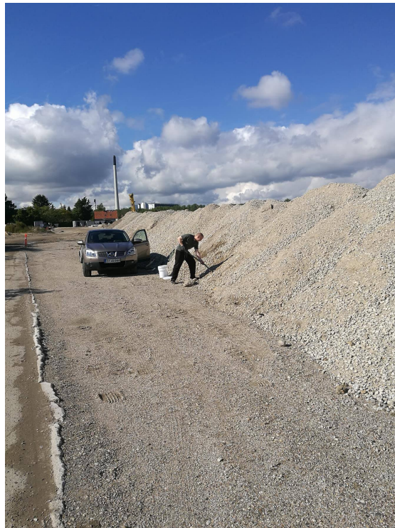
Figure 4.1: Collecting of the crushed concrete.
