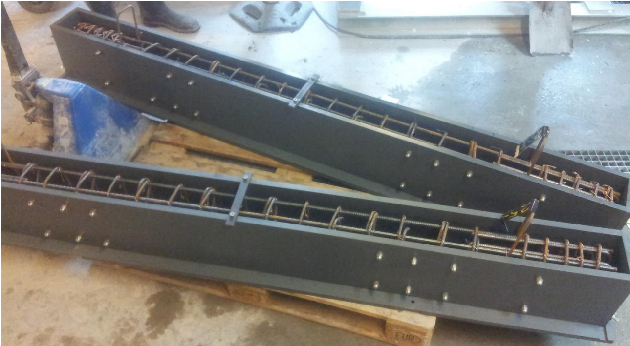
Figure 4-3: Beam and column molds, with reinforcement cages.
