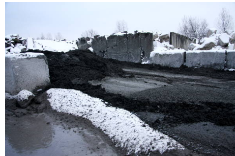
(b) Fresh concrete waste at RGS 90
